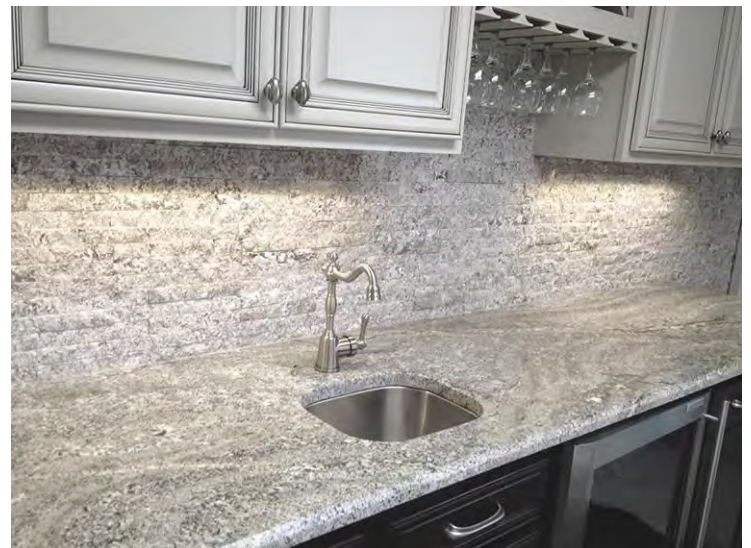
Left: This split-stone veneer wall is approximately 6 lbs. per sf., so there was no need for metal lath or grout. Right: Over 200 lbs. of white antique granite were dry-stacked in this backsplash and did not require any grout. The granite pieces are the cutoffs from the fabrication process and were split by people with special needs, through a program Recycled Granite calls Green Abilities, which creates jobs for people with disabilities. Photos courtesy of RecycledGranite.com
