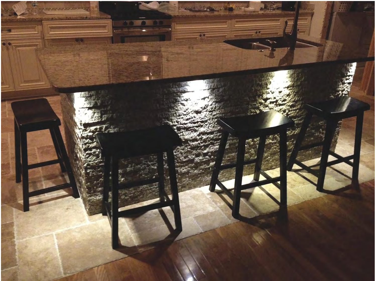
The lower part of this breakfast bar is an example of many projects that include recycled split-stone veneer. The stones can be dry stacked directly over a variety of surfaces including drywall, brick, cement board, etc. Photo courtesy of RecycledGranite.com
