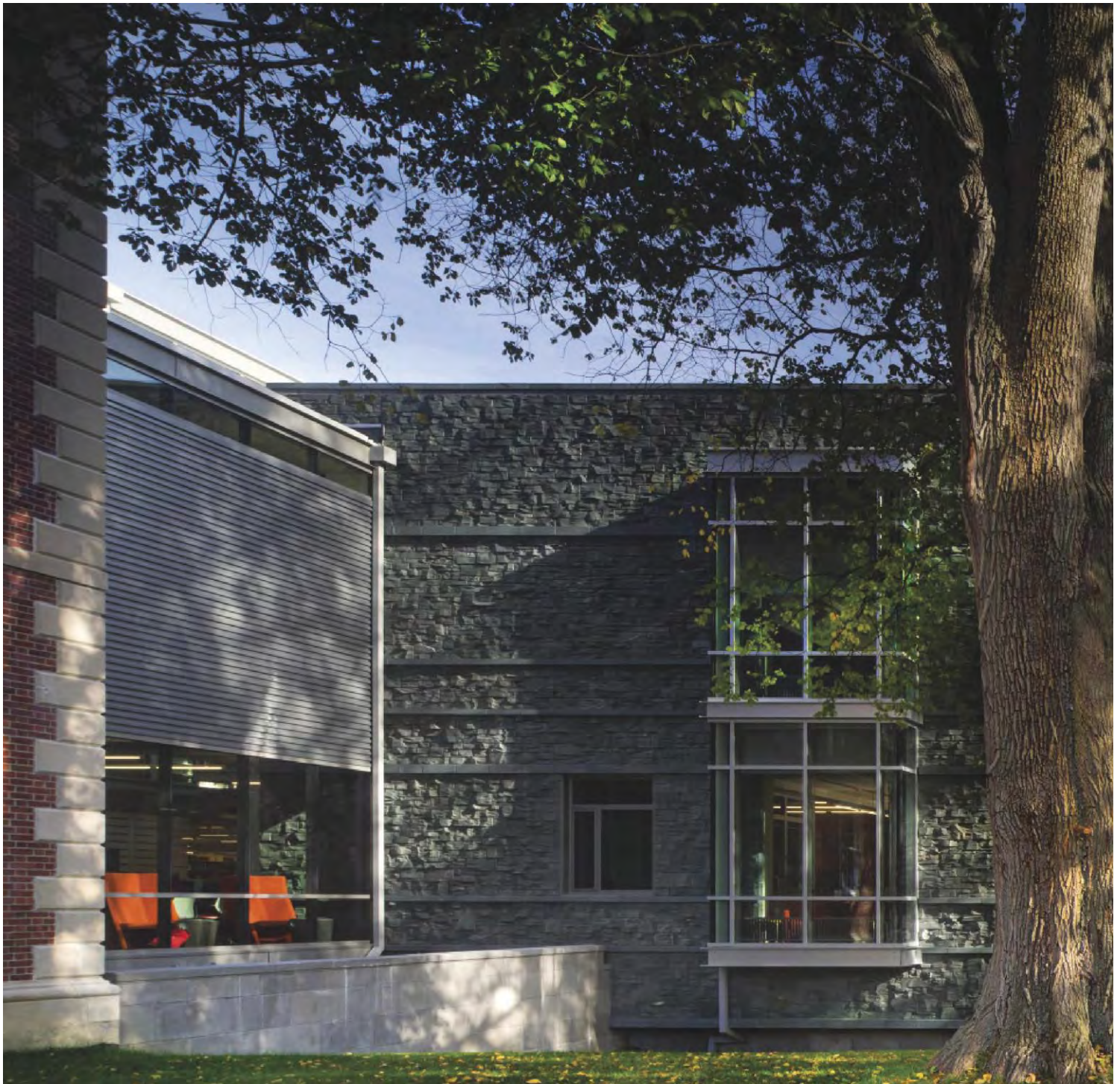
On one of the restored facades, the irregular texture of the sculpings is distinguished with the smooth, honed bands of slate. Photo © Nic Lehoux
