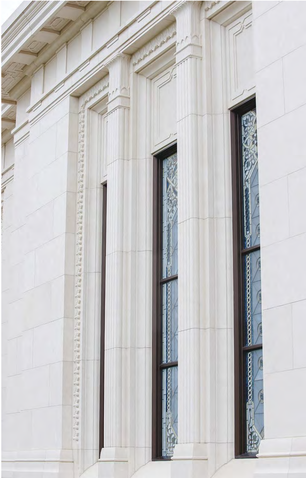
Fluted limestone pilasters were incorporated between the exterior windows. Photo © Antonio Chapital
