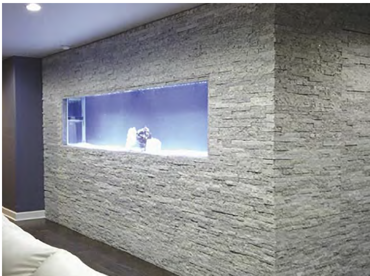
Left: This split-stone veneer wall is approximately 6 lbs. per sf., so there was no need for metal lath or grout. Right: Over 200 lbs. of white antique granite were dry-stacked in this backsplash and did not require any grout. The granite pieces are the cutoffs from the fabrication process and were split by people with special needs, through a program Recycled Granite calls Green Abilities, which creates jobs for people with disabilities. Photos courtesy of RecycledGranite.com
