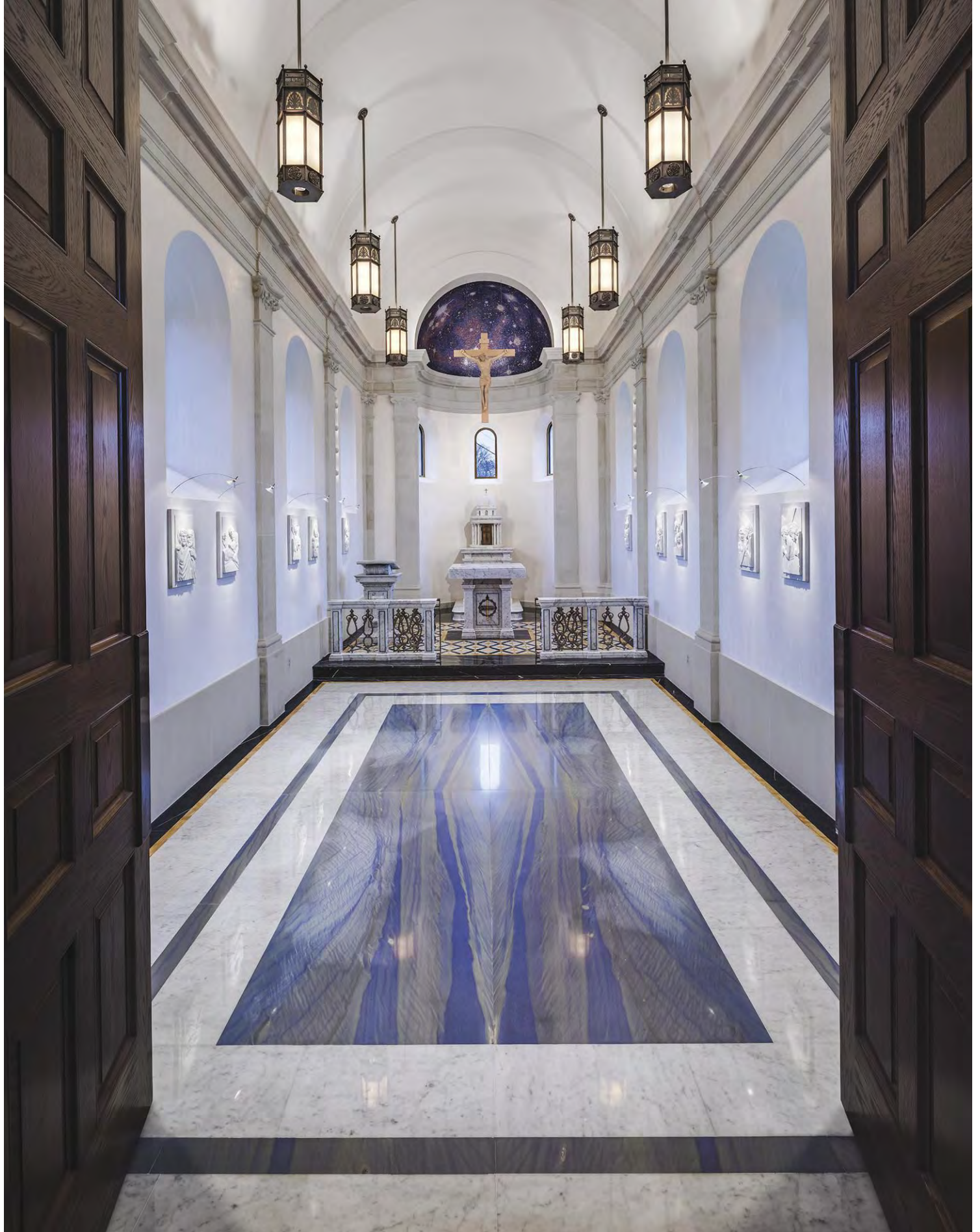
In the nave, four large slabs of Azul Macauba are arranged in a diamond book-matched pattern.
