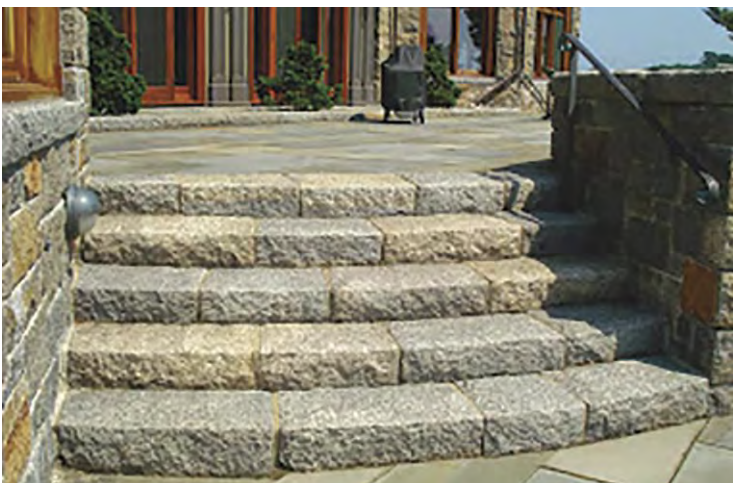
Recycled stone step installations varying in design, number and complexity. Photos courtesy of Stone Farm Living.
