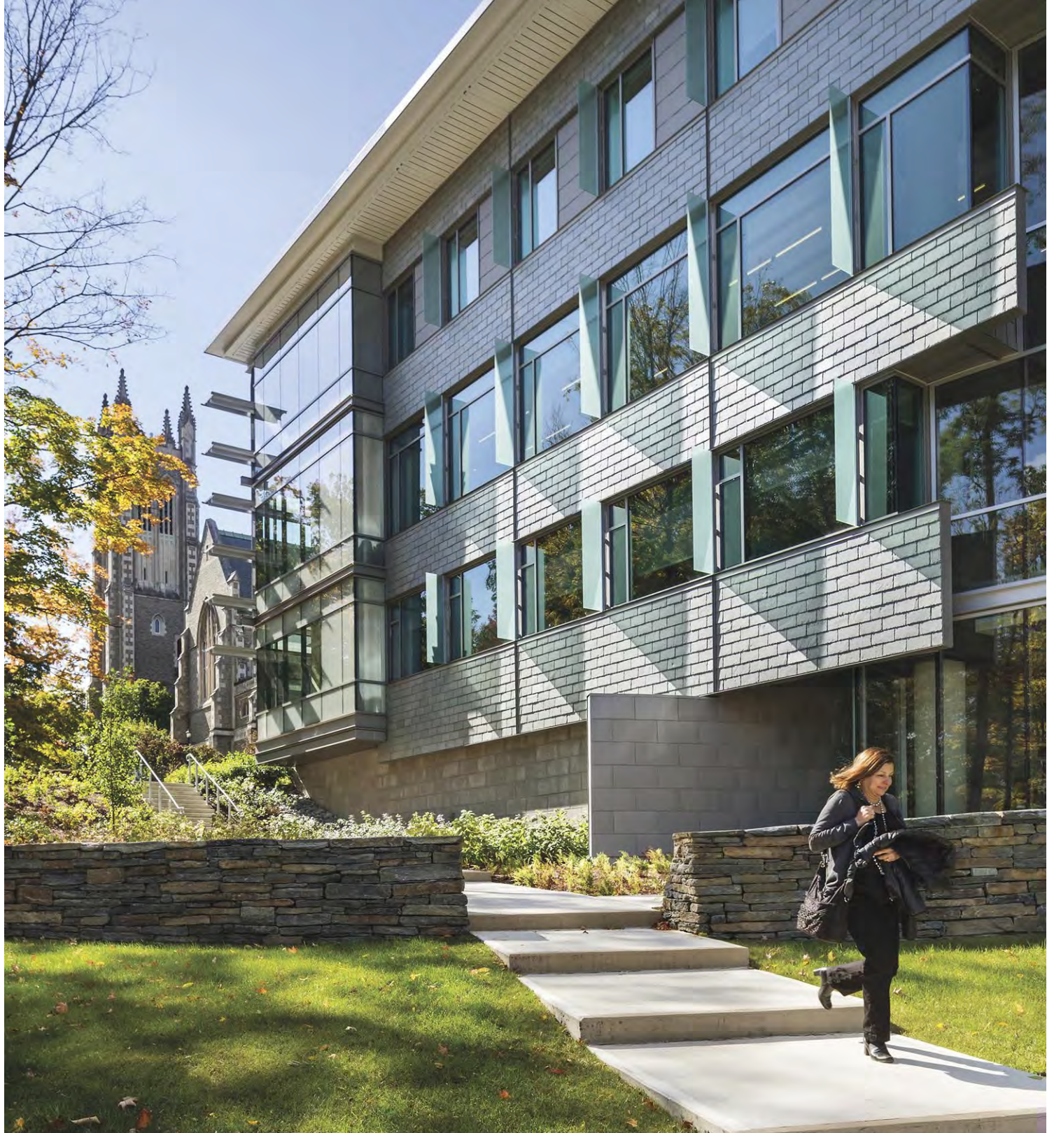
The south half of the east elevation features vertical, translucent fins, which provide some shaded relief from the daytime sunlight. The triangular shadows cast by the fins create an interesting complement on the slate wall shingles. Photo © Peter Aaron, Esto
